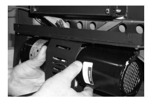
11) Mount the blower assembly in position under the base of the stove and secure with the 2 supplied bolts (2-1/4" #20 hex head)
